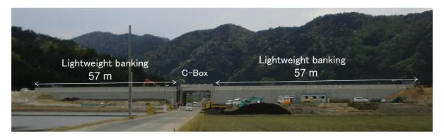
Figure 8. Lightweight banking near culvert box (STA498, taken in 2013, Tashiro et al., 2015).
