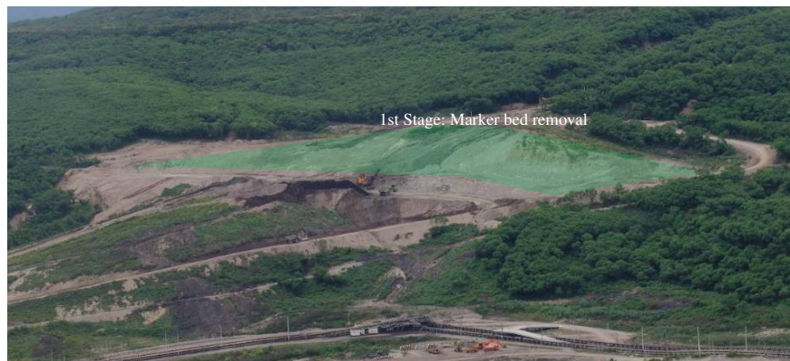
(a) Access road and Marker bed removal in 1 st Stage (as of August 2011)
