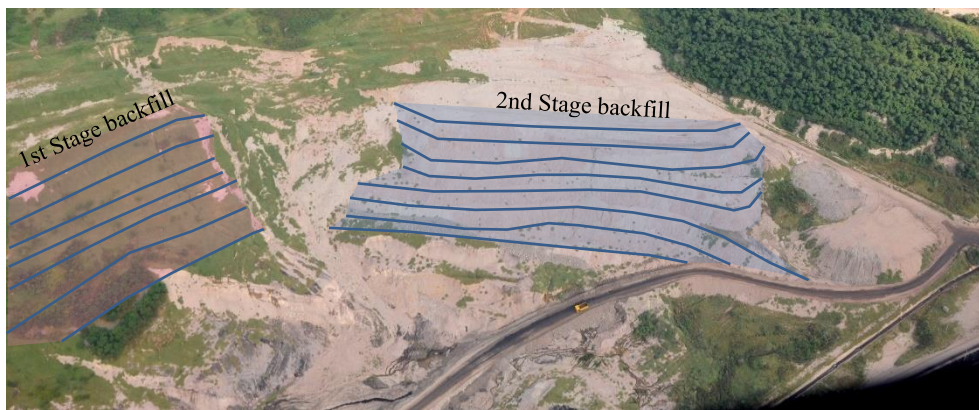
(d) Aerial view at end of 2 nd Stage (as of October 2017)
