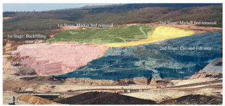
(c) Marker bed removal and 2<sup>nd</sup> Stage preparation in 1<sup>st</sup> Stage (as of April 2014)
