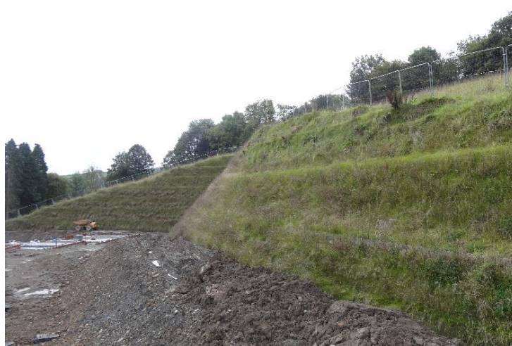
Figure 3. Vegetated structure constructed from draining geogrid and site won fill, Palmerston Park, Devon, Summer 2017.
