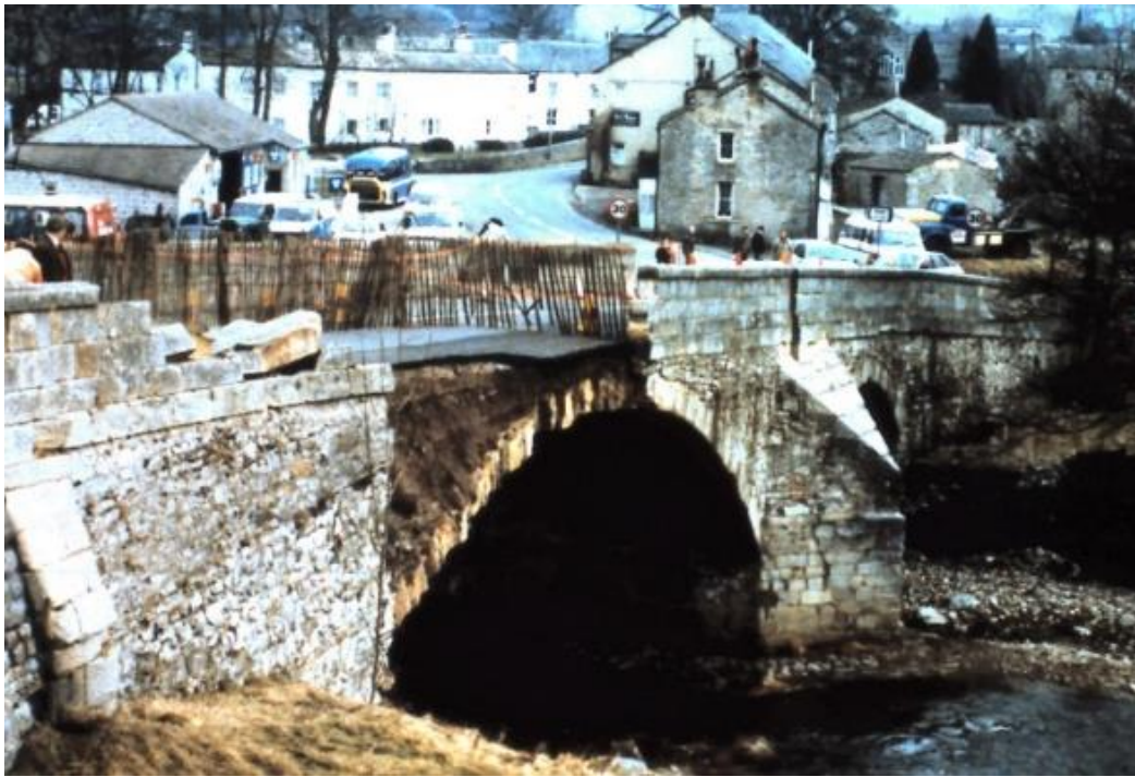
Figure 9. Failure of spandrel wall, Kettlewell New Bridge, 1984.
