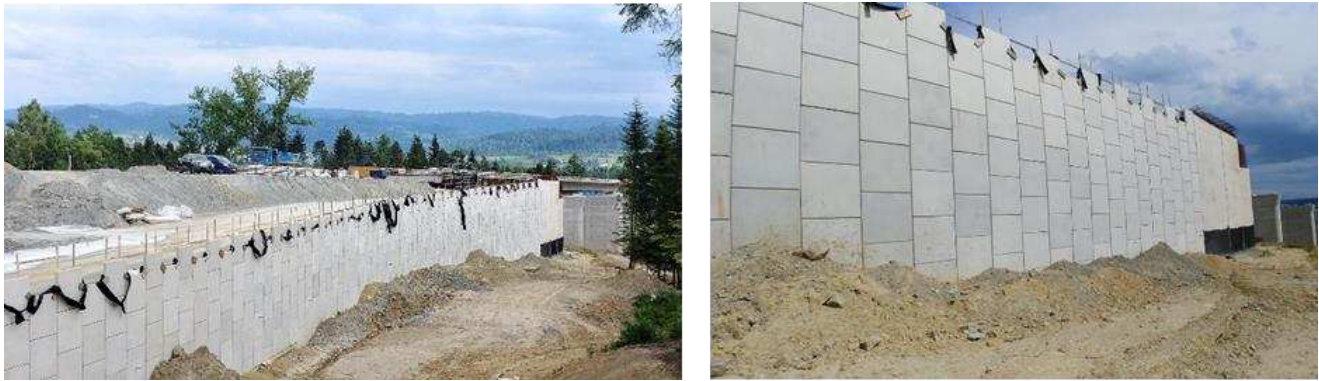
Figure 2. MSE bridge approaching ramp elevation view during construction.
