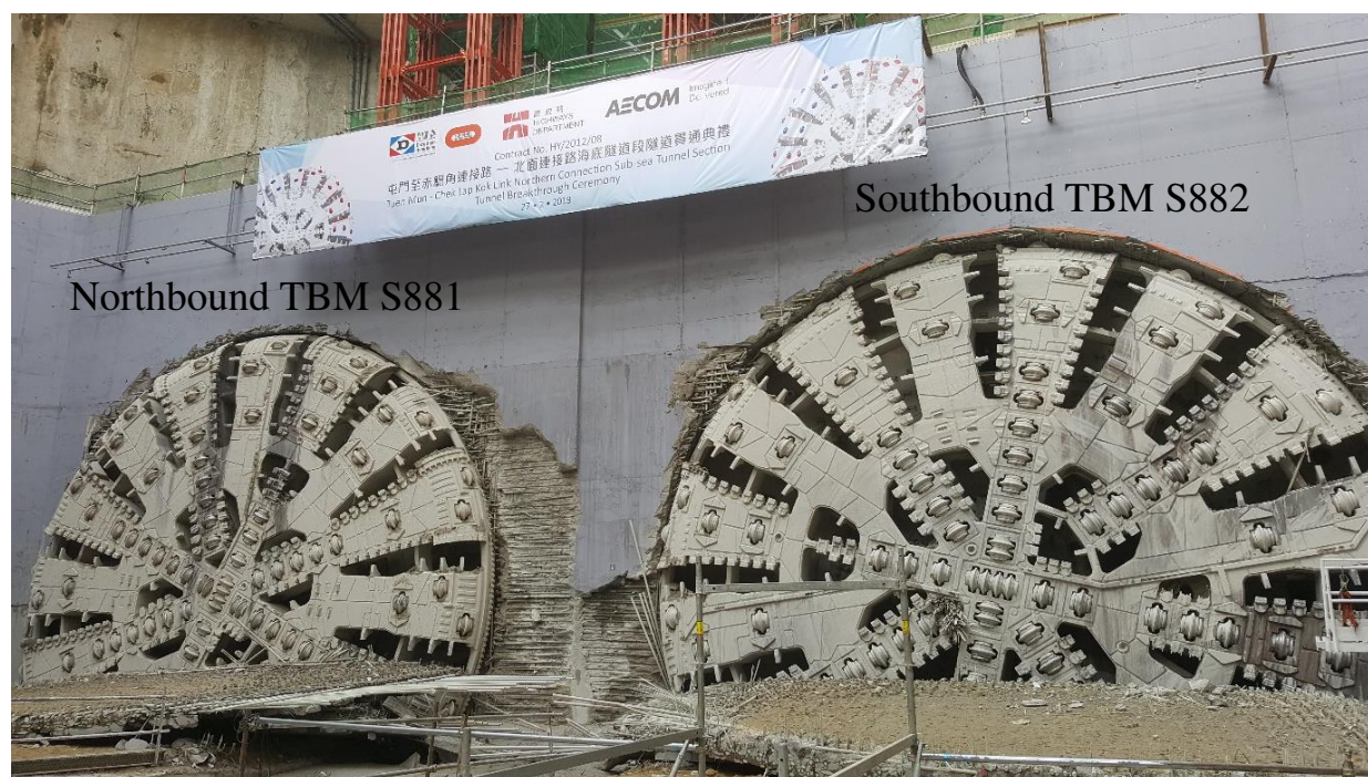
Figure 9. 14 m diameter slurry mix-shield TBMs.
