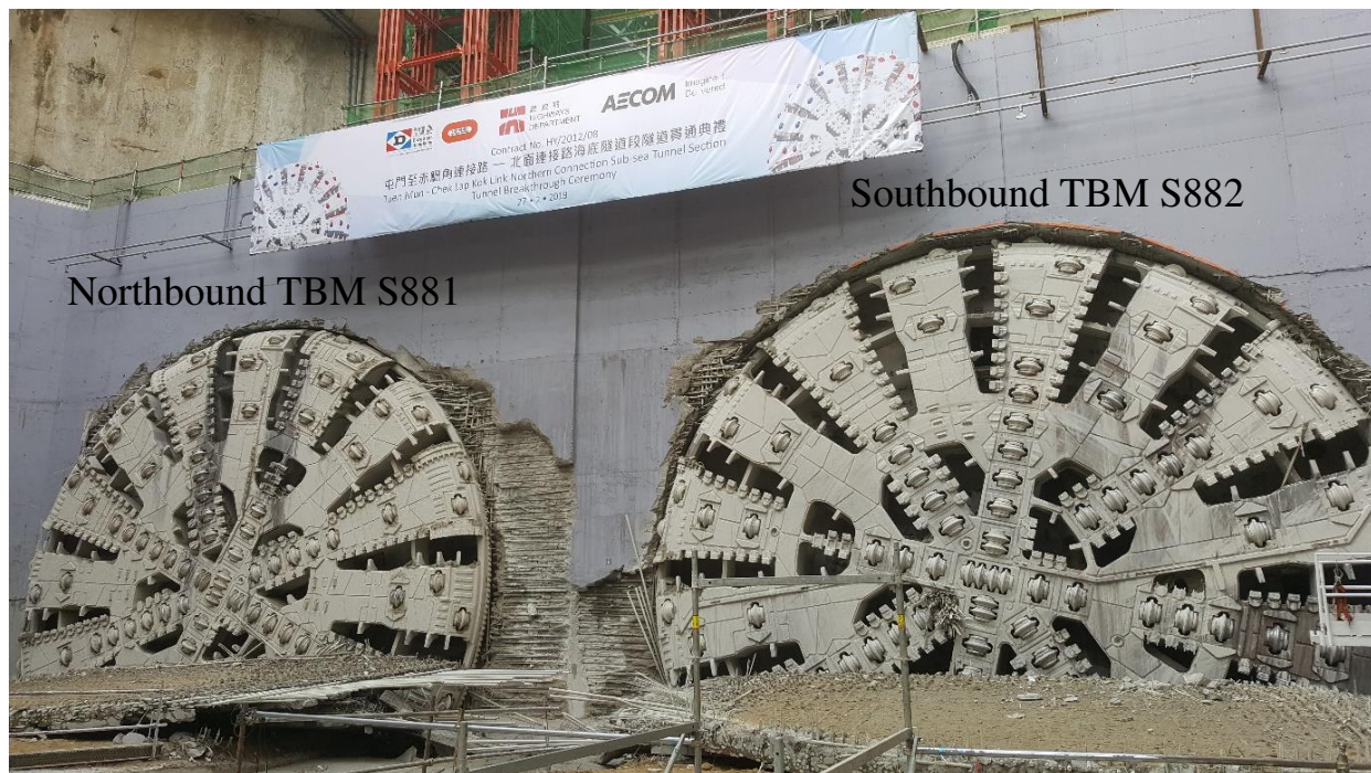
Figure 9. 14 m diameter slurry mix-shield TBMs.
