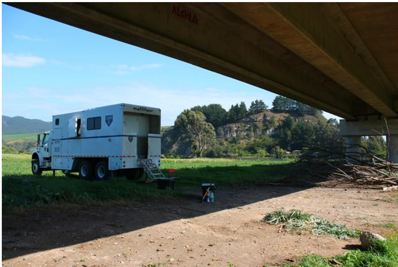
Figure 6. Photo of the north side after the 2019 earthquake (October 17 th , 2019). The CPT truck is shown here doing subsurface testing.
