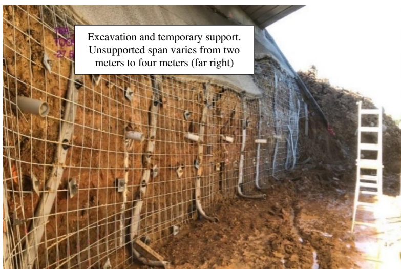
Figure 6. Excavation completed to formation level. The abutment is supported with percussion anchors and reinforced shotcrete. Note larger unsupported span on the far right.
