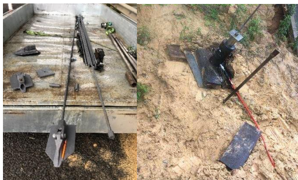
Figure 5. Percussion anchor (180-millimeter head) and load testing.
