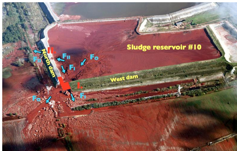
Figure 11. Based on the created flow channels in the red sludge, the flow directions were reconstructed. The initial flows F_1 and F_2 occurred at Locations I and II, pointing toward the direction of the existing fractures. The direction of flow F_1 changed to F_0 when the western part of the North dam had been washed away, creating a big opening. (Source: https://www.ndtv.com/world-news/hungarys-toxic-sludge-spill-as-big-as-gulf-oil-leak-435094 .)
