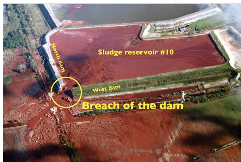
Figure 2. Aerial photo of the breach of the tailing dam. (Source: https://www.ndtv.com/world-news/hungarys-toxic-sludge-spill-as-big-as-gulf-oil-leak-435094 .)
