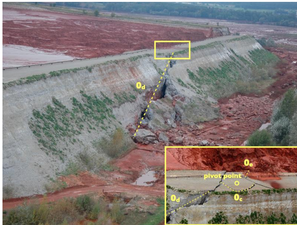
Figure 15. Shear fractures ( 0_c and 0_d ) caused by compressional stress at Location II are shown. These fractures were formed at the breach, resulting from the angular distortion of the failed dam section. On the opposite (reservoir) side, at the same time, extension fracture 0_e occurred (Figure 9), extending the existing fracture of -2_b . (Sources: https://www.nbcnews.com/slideshow/toxic-red-sludge-floods-towns-near-budapest-39514793 ; http://www.hungarianambiance.com/2011/09/possibility-of-act-of-terrorism-cant-be.html ).
