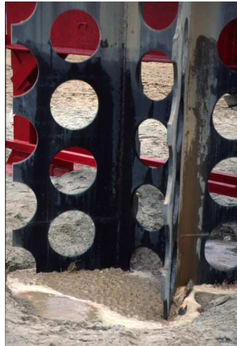
b) Liquefaction during DVVCR
