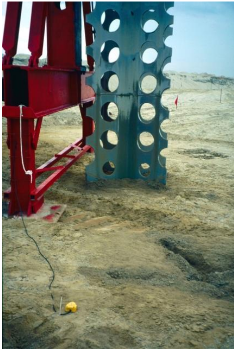
a) Triaxial geophone located at 6 m distance from the compaction probe
