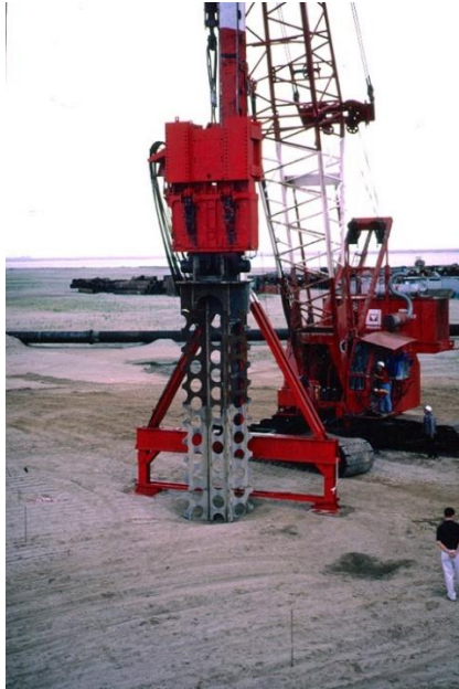
a) Vibrator clamped to flexible compaction probe.
