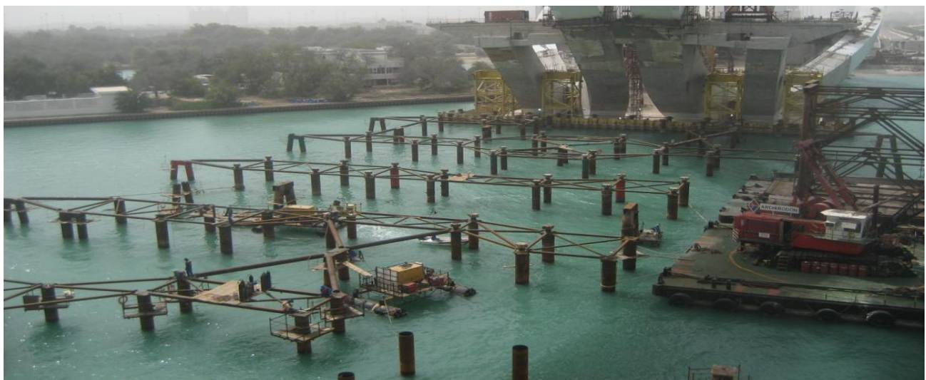
Figure 2. Driving of Temporary Piles and Welding of Bracing.
