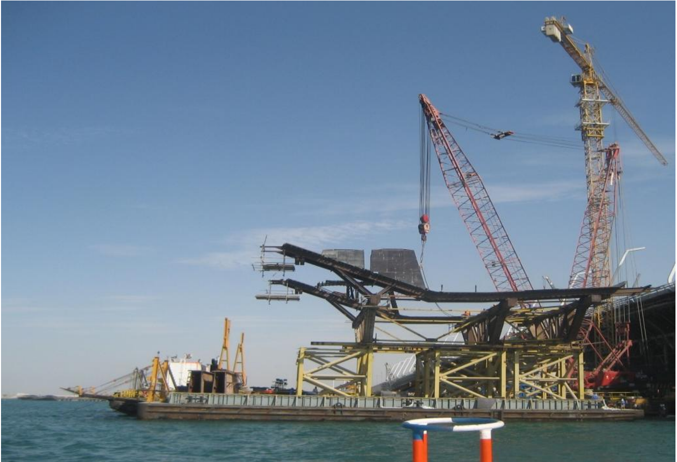
Figure 3. Falsework Lowered onto a Barge.
