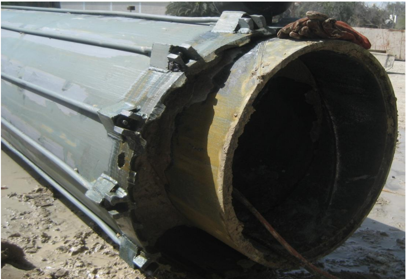
Figure 14. Extraction of the casing pile along with the existing pile.
