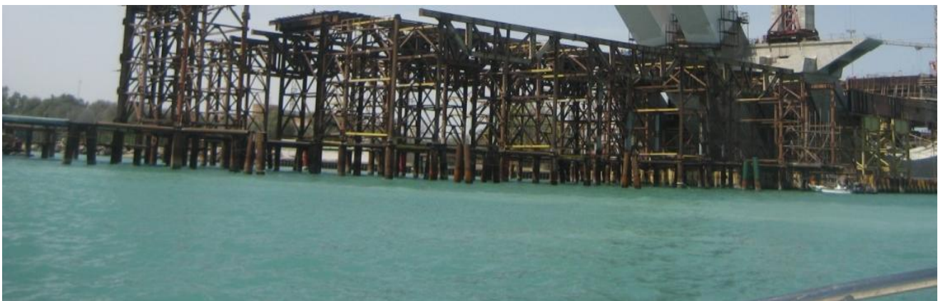
Figure 1. Temporary works – Falsework Erection on Piles.
