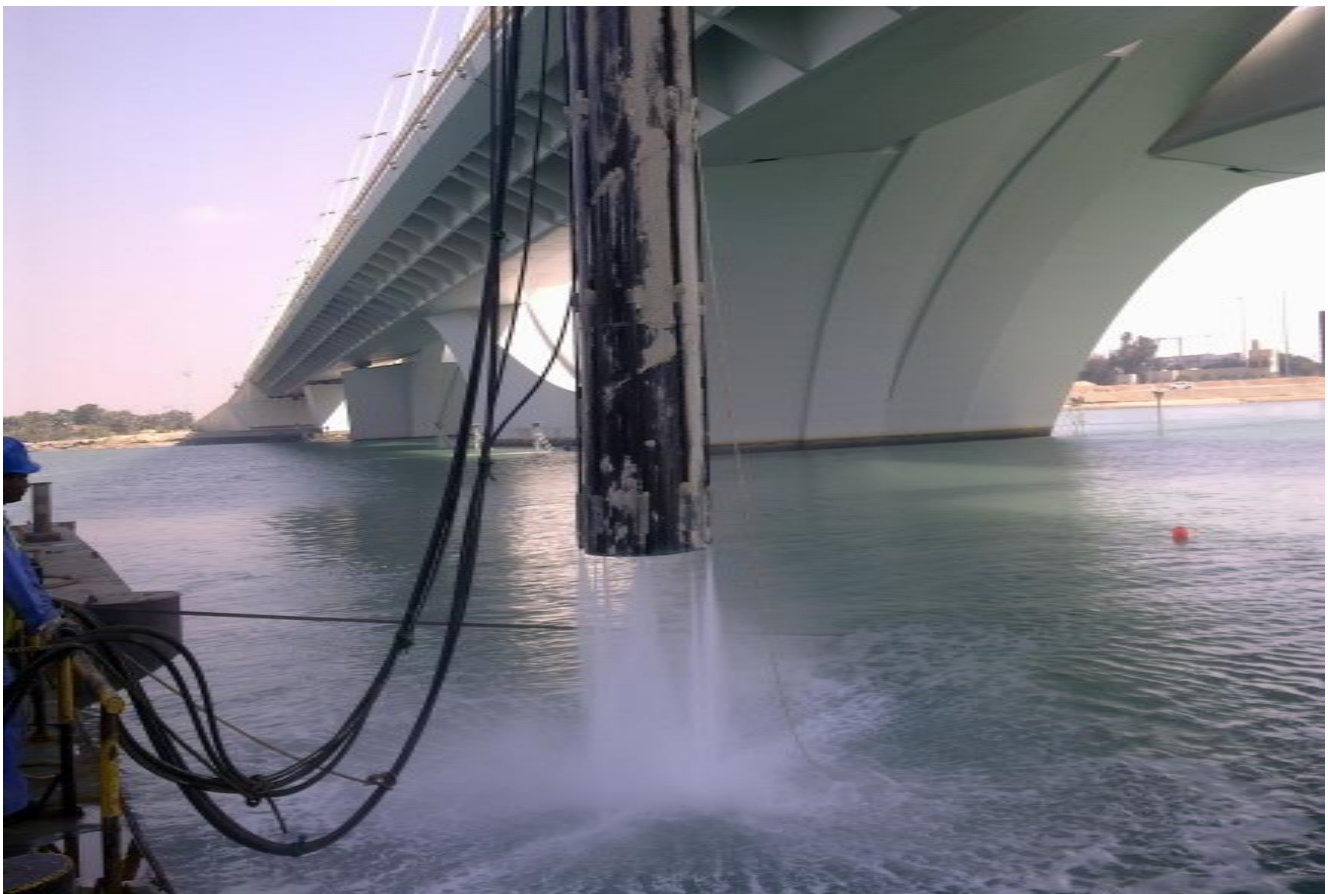
Figure 7. Water Jet Method - Casing Pile.
