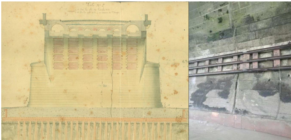
Figure 4. Fracture on P02, illustrated on the left (1860, departmental archives) and pictured on the right (2014).
