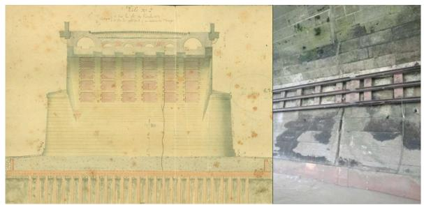
Figure 4. Fracture on P02, illustrated on the left (1860, departmental archives) and pictured on the right (2014).
