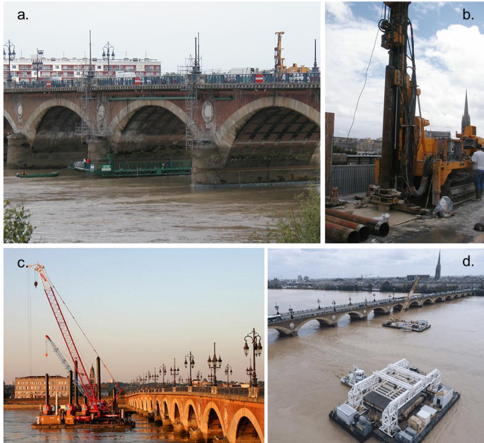
Figure 6. Illustration of works: (a) Post-tensioning on P05 and P06, (b) Micropiles on P05 and P06, (c) driven dolphins works on P08 and P09 (source: Bernard Tocheport), (d) rip-rap works on whole bridge (source: Sud-Ouest).
