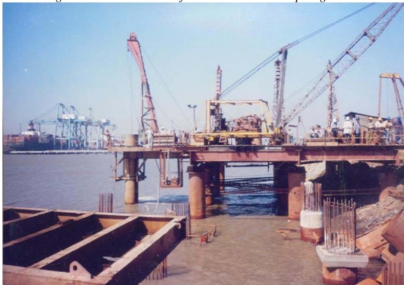
Figure 11. Construction of Piles.
