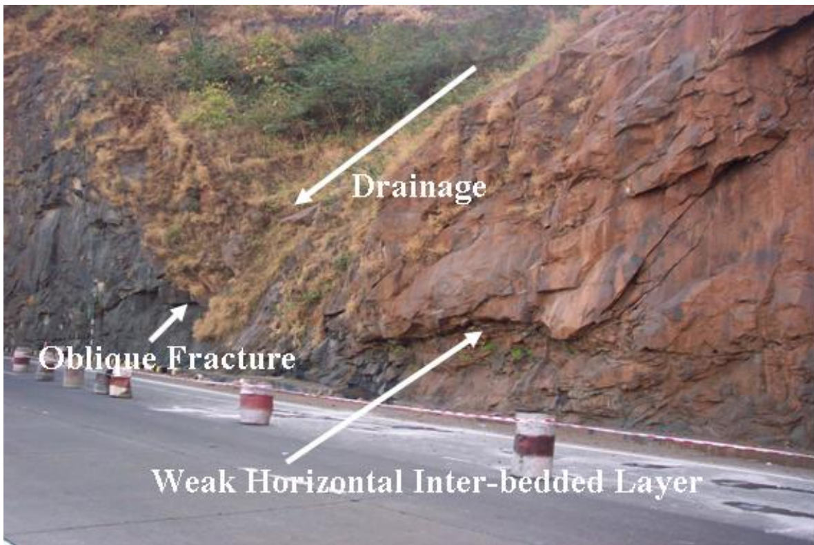
Figure 6. Intersection of oblique and sub-horizontal fractures.
