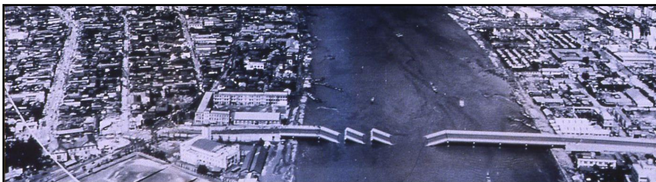
Figure 1. Collapse of Showa Bridge.
