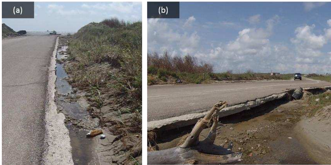
Figure 4. (a) Road undermining due to erosion and scour was observed on both sides of East Cotter Avenue, and (b) a 0.4 m undercut was measured at the beginning of a newly formed breach (collected September 3, 2017; location 27°50'8.53"N, 97°2'55.00"W).
