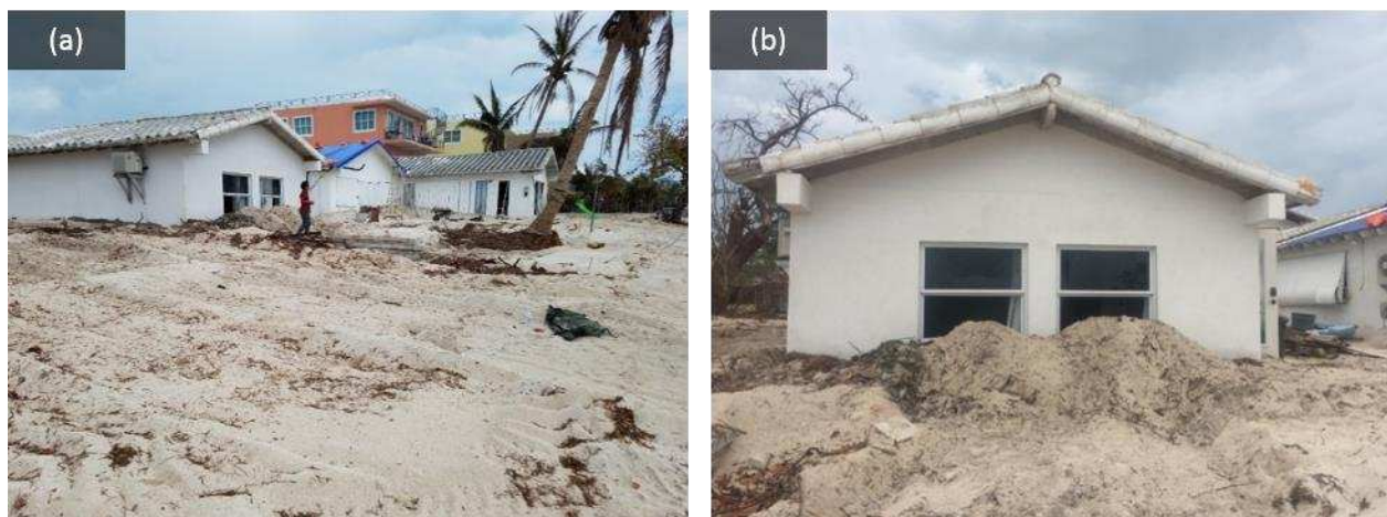
Figure 13. (a) Large volumes of sediment were deposited around houses and other structures and (b) buried them with approximately 1 m of sand, reaching the bottom of window sills (collected September 26, 2017; location 24^{\circ}41'31.52''\text{N} , 81^{\circ}4'56.31''\text{W} ).
