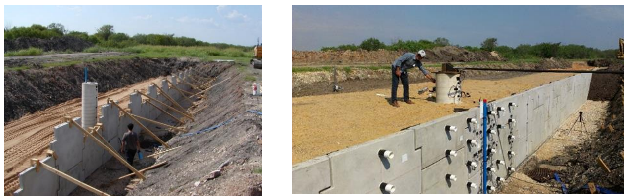
Figure 30. Construction of the MSE wall.
