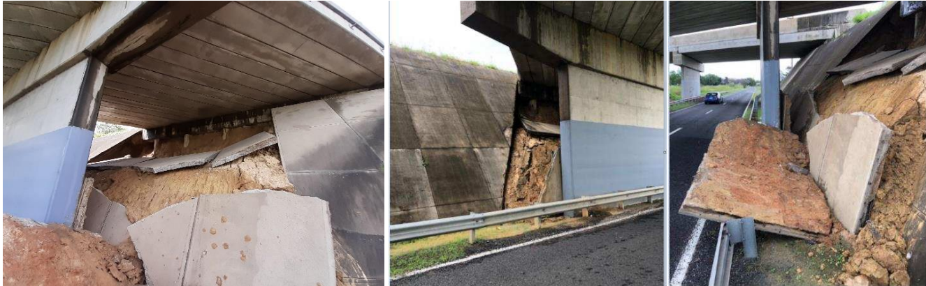
Figure 2. Abutment condition after failure.
