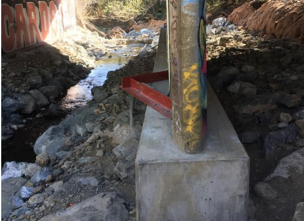
Figure 12. Closeup looking downstream at Pier 3 sonar device.
