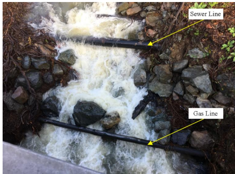
Figure 1. Looking upstream from the existing bridge at the undermined pipes (January 2017).
