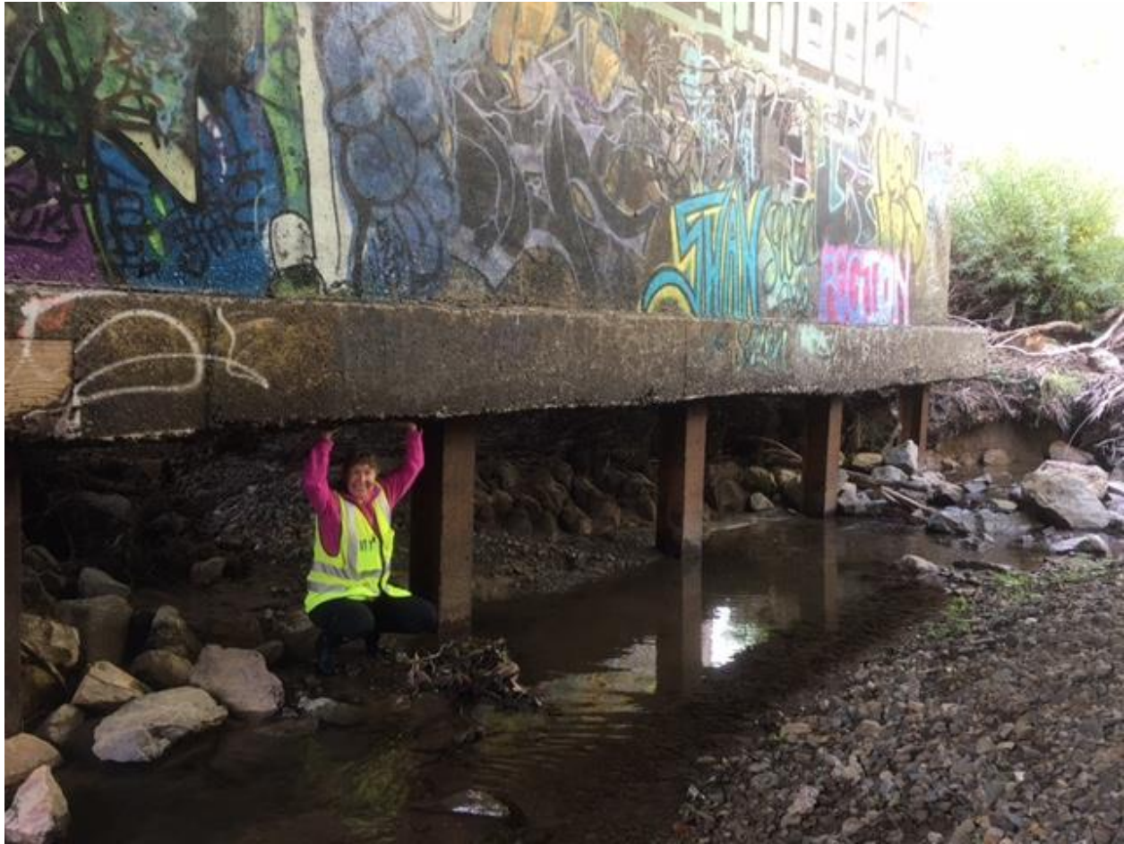
Figure 4. Looking upstream at Pier 3 pile exposure with author (November 2017).
