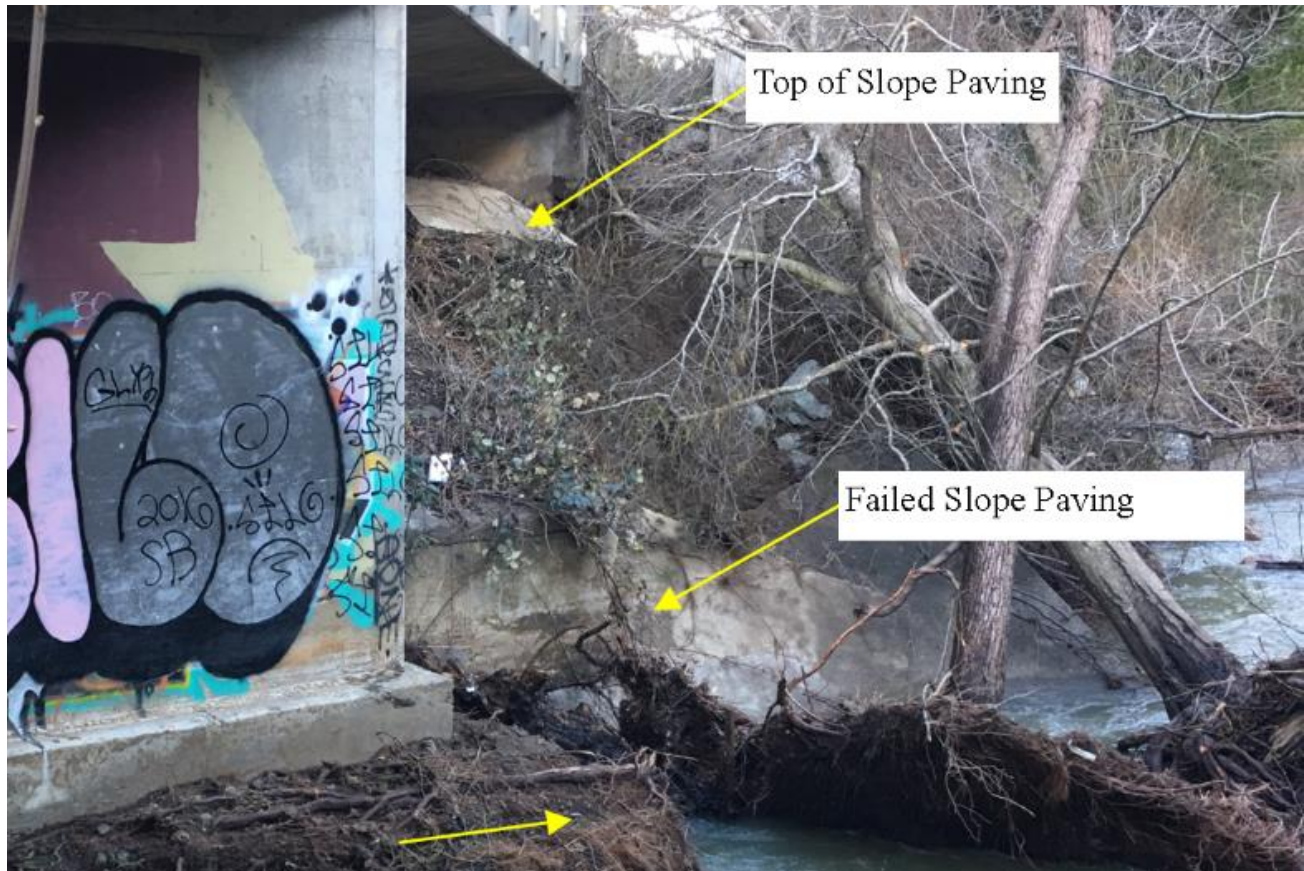
Figure 5. Slope paving at Abutment 5, which is undermined and has fallen into the creek.
