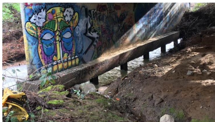
Figure 3. Upstream of head cut looking at Pier 3. Approximately 0.6 to 1 meter of pile are exposed below the bottom of the footing.
