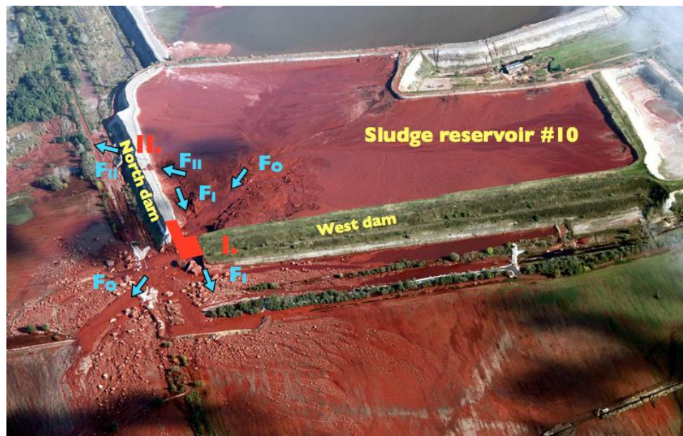
Figure 11. Based on the created flow channels in the red sludge, the flow directions were reconstructed. The initial flows F_1 and F_2 occurred at Locations I and II, pointing toward the direction of the existing fractures.
