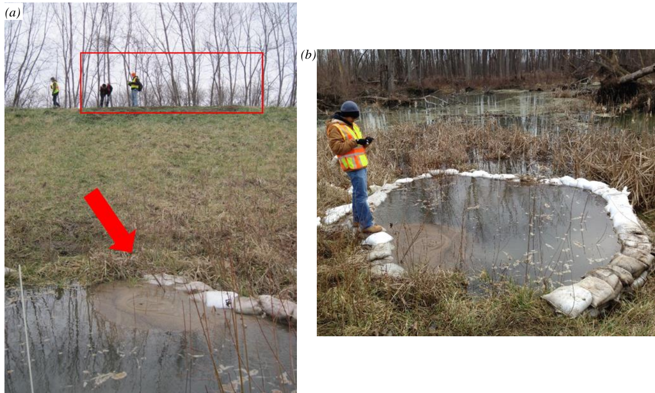
Figure 5. December 2015 flood reconnaissance: (a) settlement of crown with active sand boil at toe of levee, (b) active sand boil with sand bag ring (Rutherford et al. 2016).
